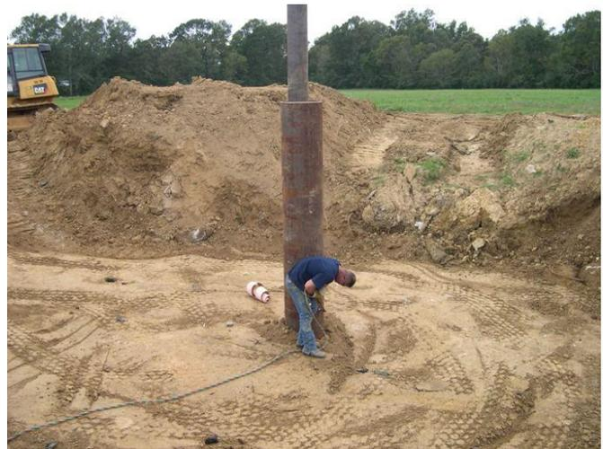
*Extension of well casing to ground level*
