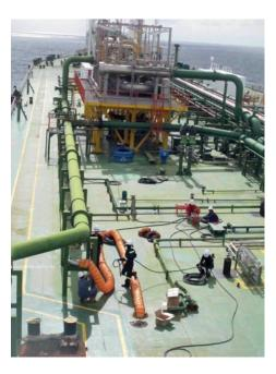
Work on the FSO was carried out above deck, administering HCD Tank Clean to the tanks below. Tank Clean successfully reliquefied sludge oil deposits in situ without the need for removal and disposal.
